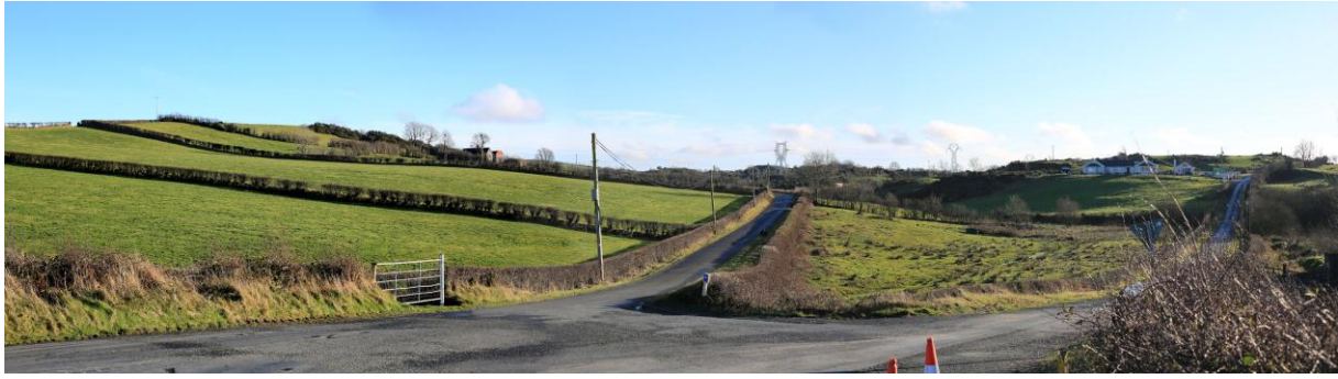
Photomontage 28 from Ouvry Cross Roads, at a distance of approximately 610m. This represents an open view between drumlins. Three towers are partly visible, travelling into the distance, others are screened by topography.
